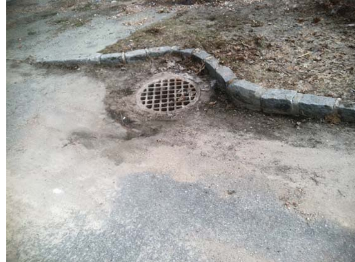
30. Stormwater catch basin at access entrance, Belgium block curbing
