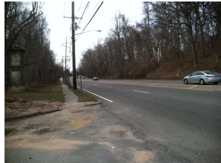
24. Searingtown Road, looking north, upslope, asphalt sidewalk, two lanes in each direction
