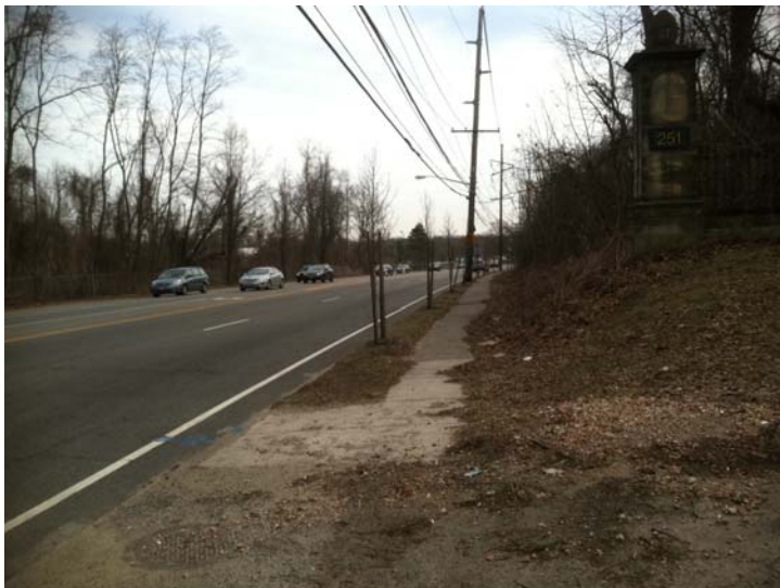
23. Searingtown Road looking south from entrance, good sight distance, asphalt sidewalk, new street trees, overhead utilities, sewer in street, traffic signal at park
