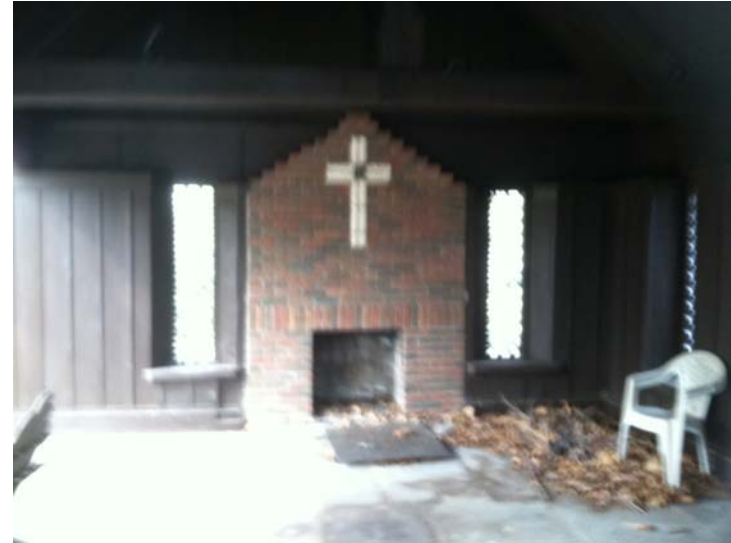
2. Fireplace inside small 1-story masonry-wood building
