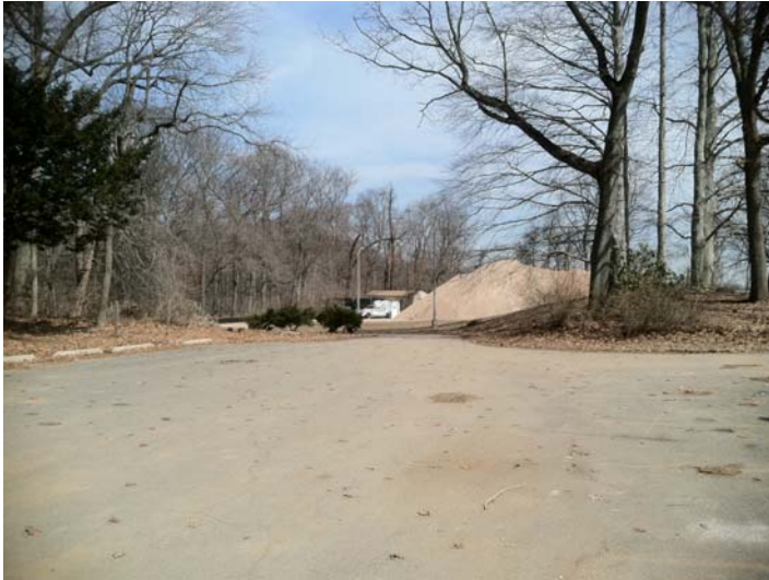
17. Looking west from parking lot toward demolition debris pile and storage shed
