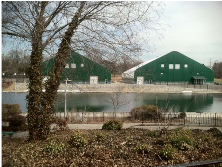
31. Christopher Morley County Park, looking east at reflecting pond and indoor tennis courts
