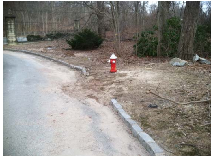
4. Looking east down paved site access, fire hydrant, Belgium block curb, water service, stormwater catch basin at end
